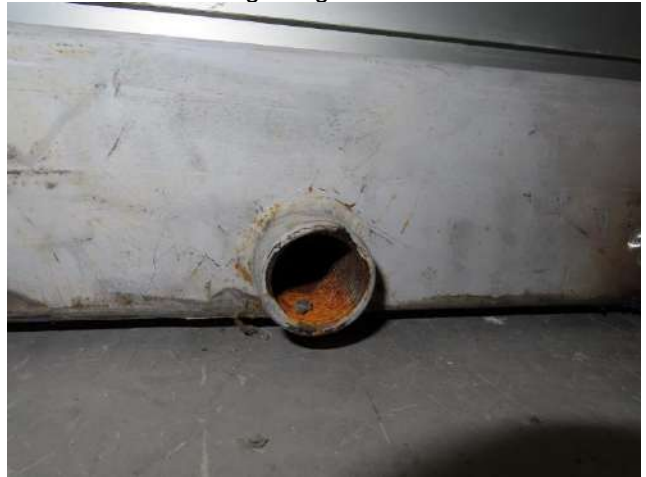
Picture 22 Drainage slot, seen from outside
