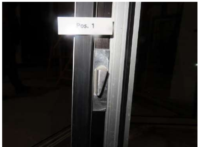
Picture 24 Locking situation 1, casement
