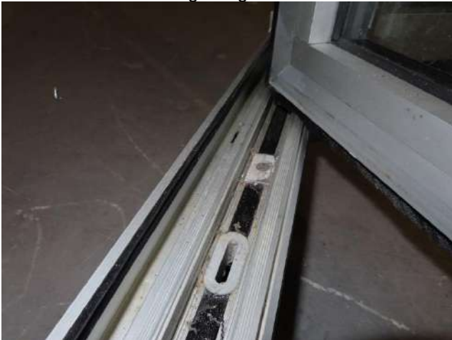
Picture 21 Frame at bottom with rebate drainage slot
