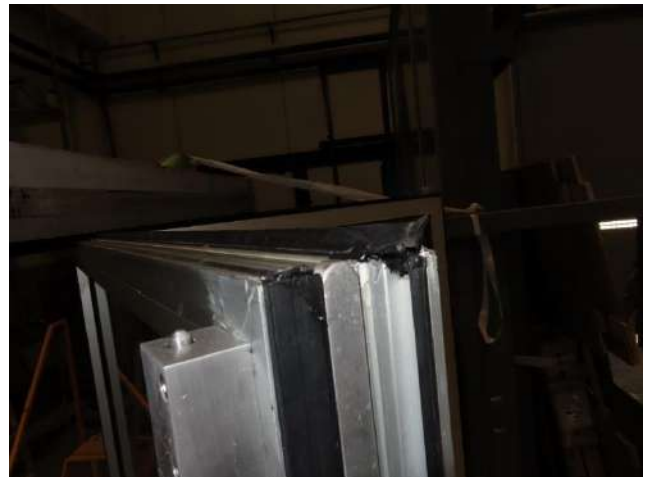
Picture 12 Casement at top
