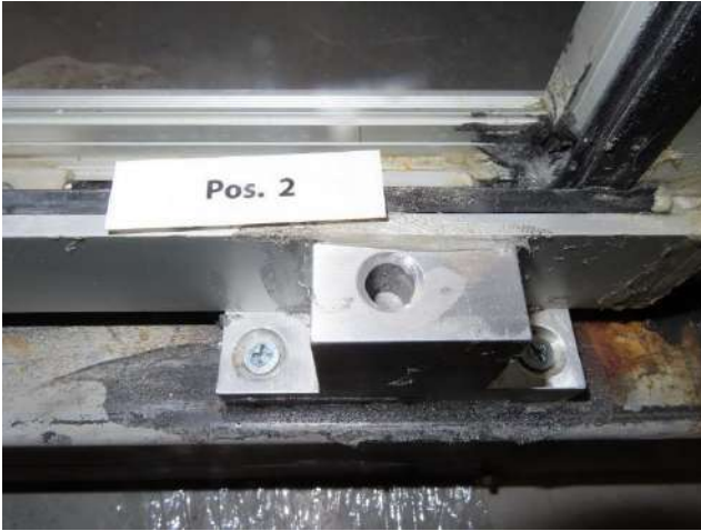
Picture 25 Locking situation 2 and 3, frame
