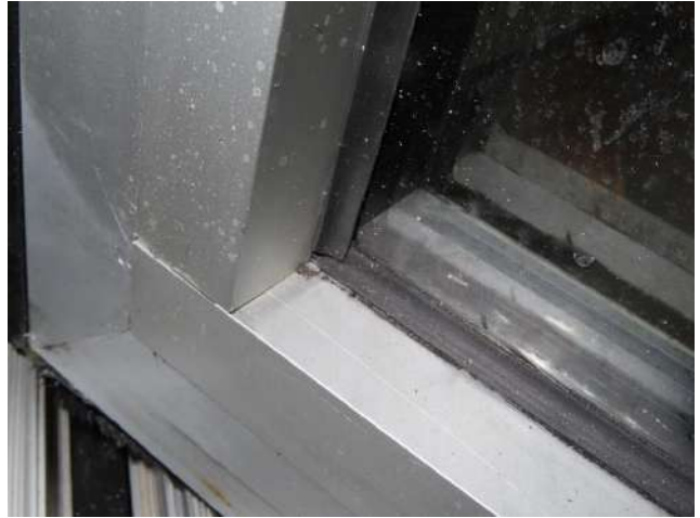
Picture 20 Internal glazing seal
