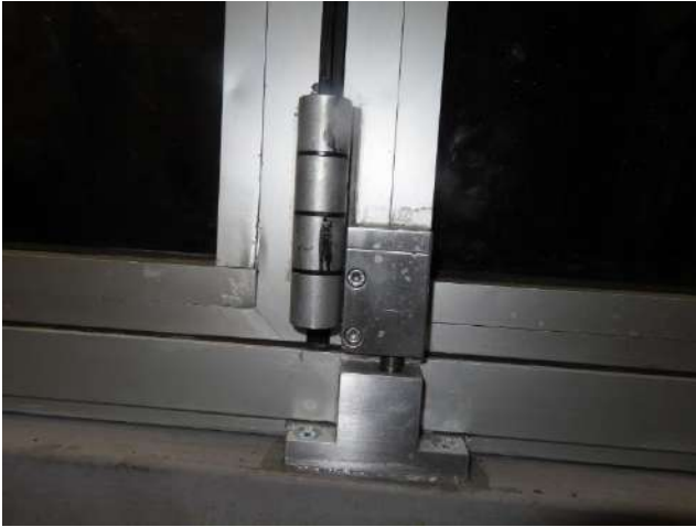
Picture 7 Hinge seen from opening side
