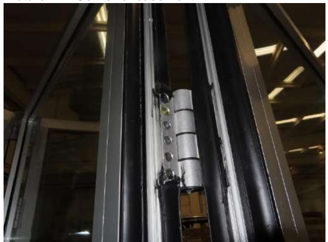
Picture 6 Hinge seen from rebate
