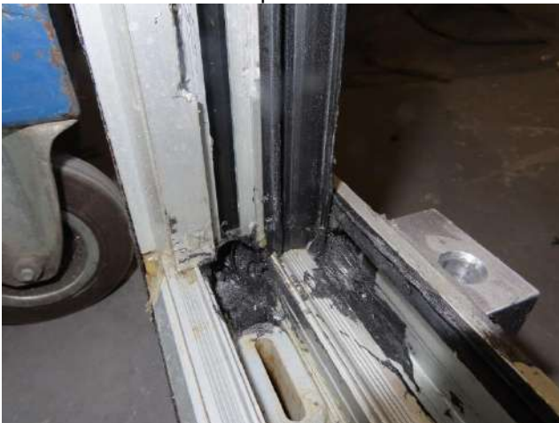
Picture 11 Frame at bottom, seen from rebate
