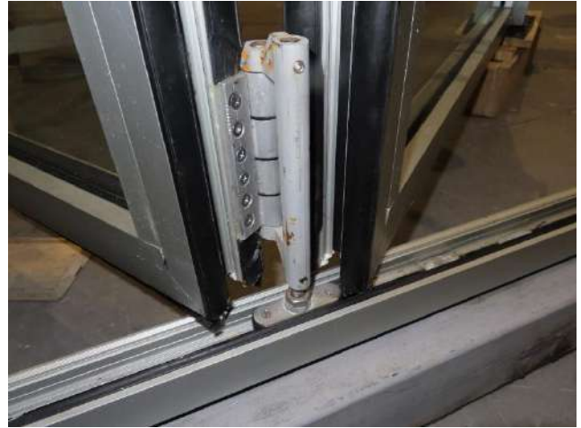
Picture 8 Hinge seen from rebate
